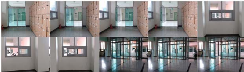
Figure 8. Images of opened/closed of door and window.
