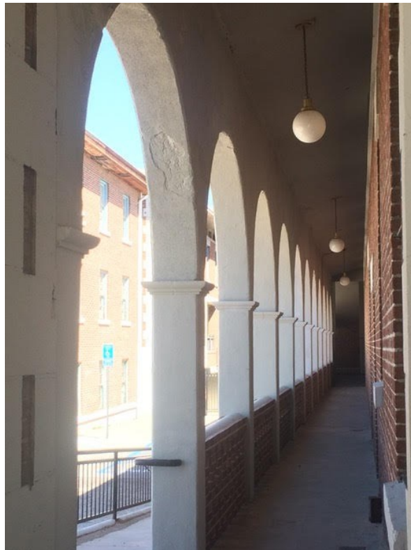
Corridor above the street
